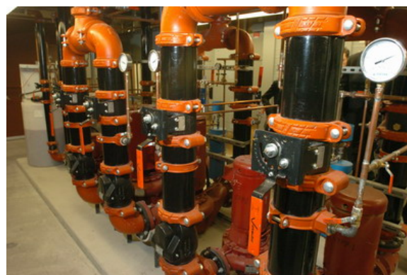
Figure 3 : Secondary fluid pumping system for heat recovery
